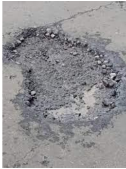
Gambar 1. Kerusakan ravelling (Hardiyatmo 2015)
